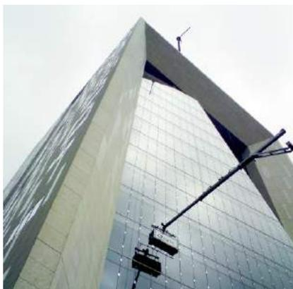
Figure 4. Example: extending cradle accessing deep recess (Source: Cox Gomy1)
